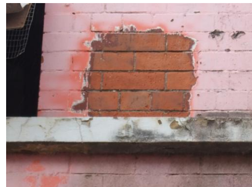
Phase I Paint Removal
