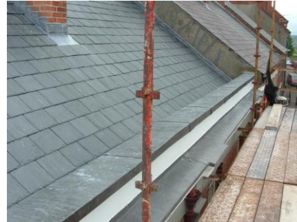
Phase I Roof Repairs
