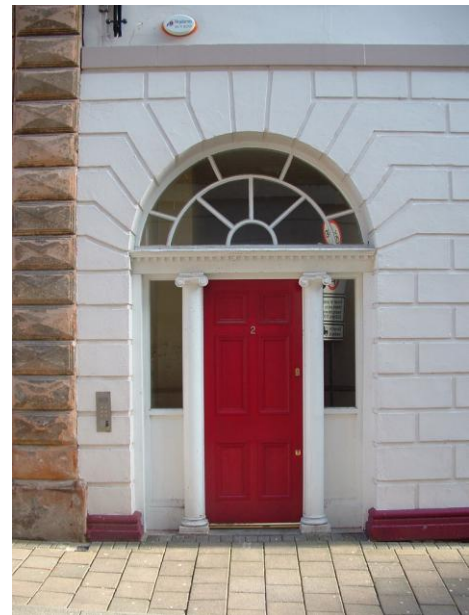
Phase I Restored Doorway
