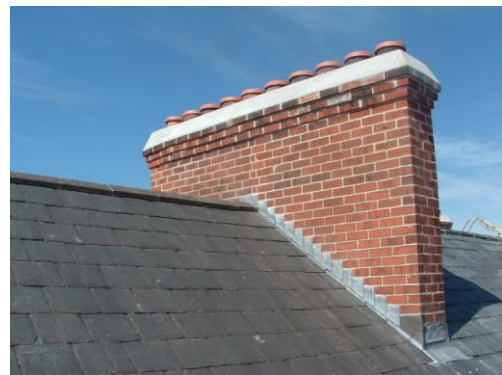
Phase I Repaired Chimney
