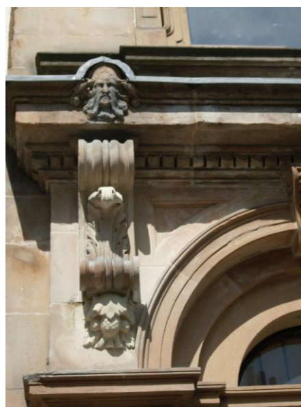
Restored Console Bracket
