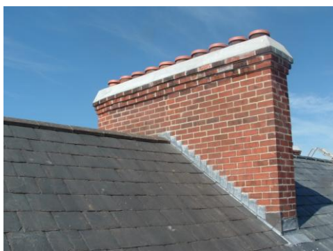
Rebuilt Chimney Stack
