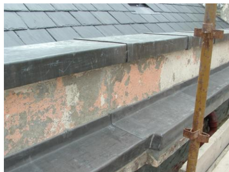
Parapet and Cornice Lead Detailing
