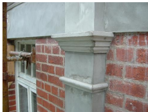
Reconstructed Pilaster Detail
