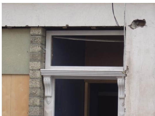
Construction of Door / Fanlight
