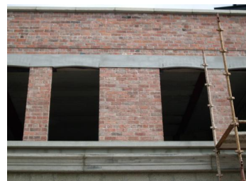
Reconstructed Salvaged Brick Panel
