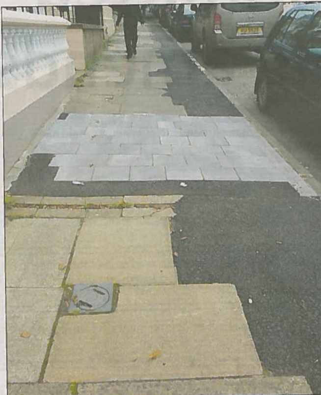
A sample of the paving at Clarendon Street.
